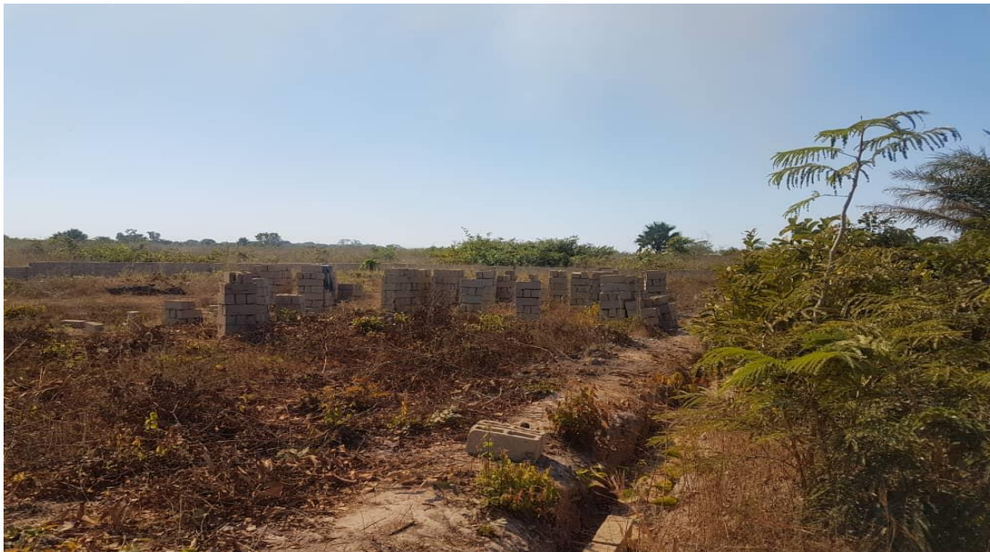
Figure 4.3: Cement-blocks packed near foundation trench to construct fence
