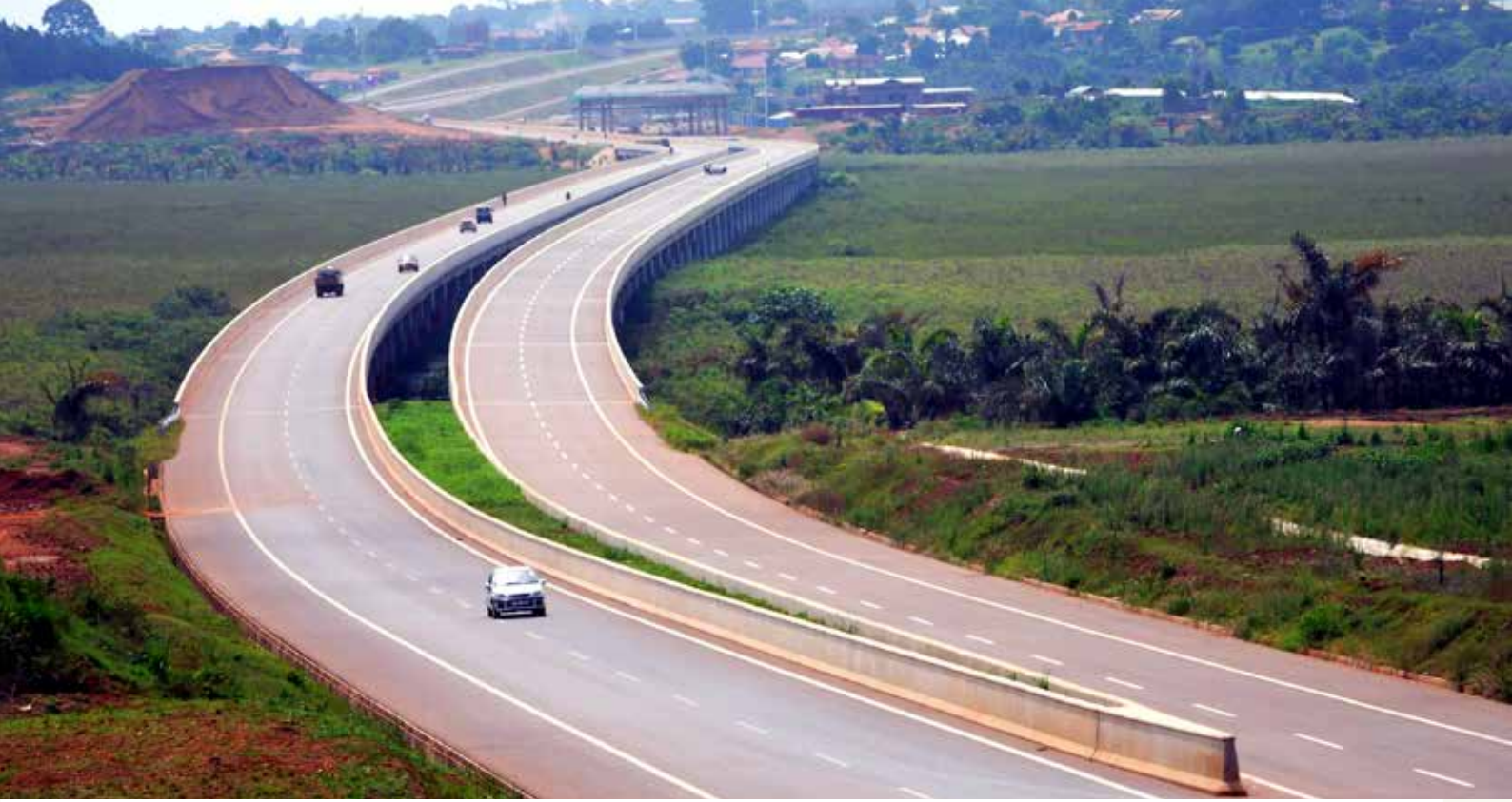
▲ Entebbe Expressway construction works (Morgan Mbabazi, 2017)
