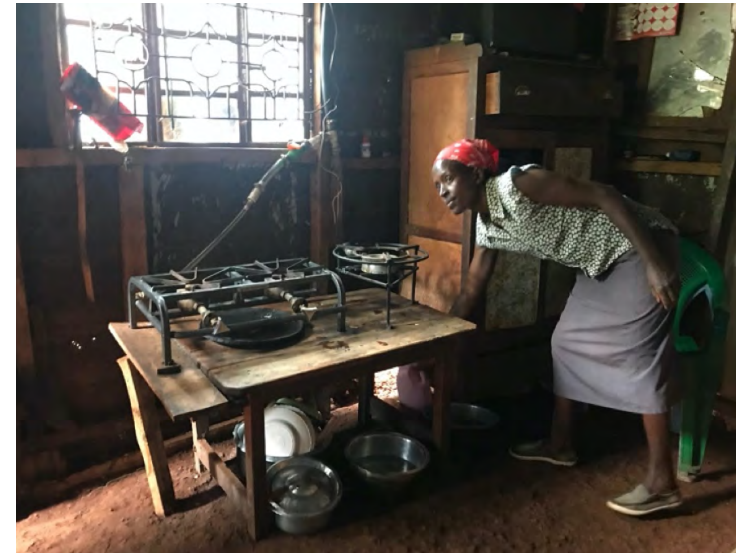
Kenyan kitchen equipped with a biogas-burning stove.
