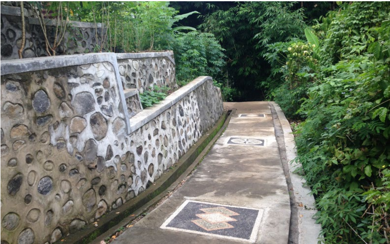
Figure 10. Road built by the community along with the landslide mitigation.
