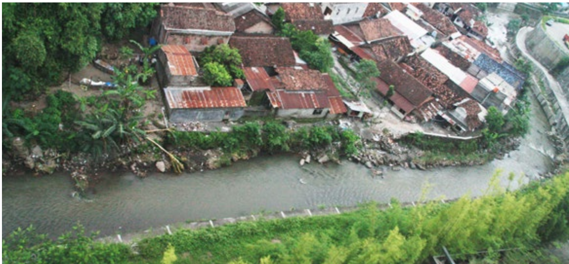
Figure 5. Flood-prone riverbank areas
