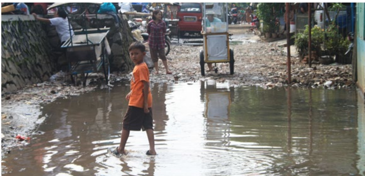
Figure 3. Road infrastructures that are not well built
