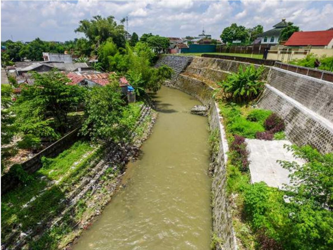
Figure 4.8 Making Gabions and River Embankment as part of Structural Mitigation along Winongo River
