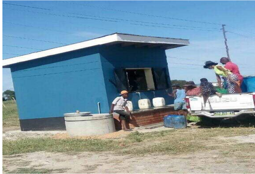
Figure 5: Water kiosk in operation
