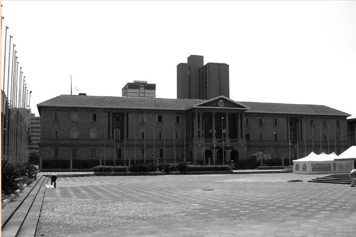
Government building in Nairobi. Photo from picasaweb.google.com .
