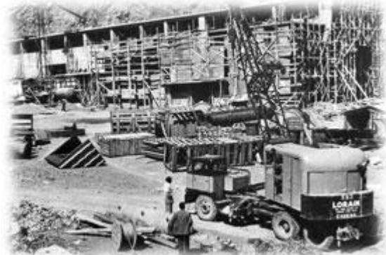
Early construction work of the Los Cipreses hydroelectric power plant
