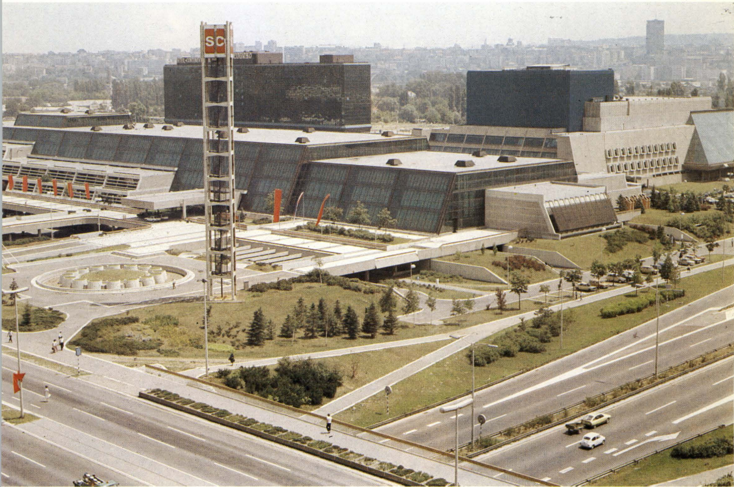
The „Sava” Congress Center in Belgrade and the „Intercontinental” hotel. All three buildings, first the conference building and then the concert and congress building and the hotel were built by „Trudbenik” in three years according to a Yugoslav design.
