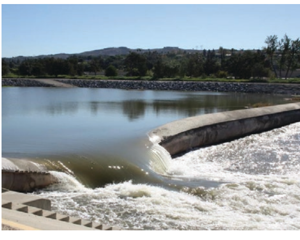
PHOTOGRAPH 3.2. Inflatable Rubber Dams Used to Maximize Groundwater Infiltration, Orange County, CA
