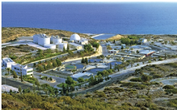
a. Limassol (moni) wastewater treatment plant
