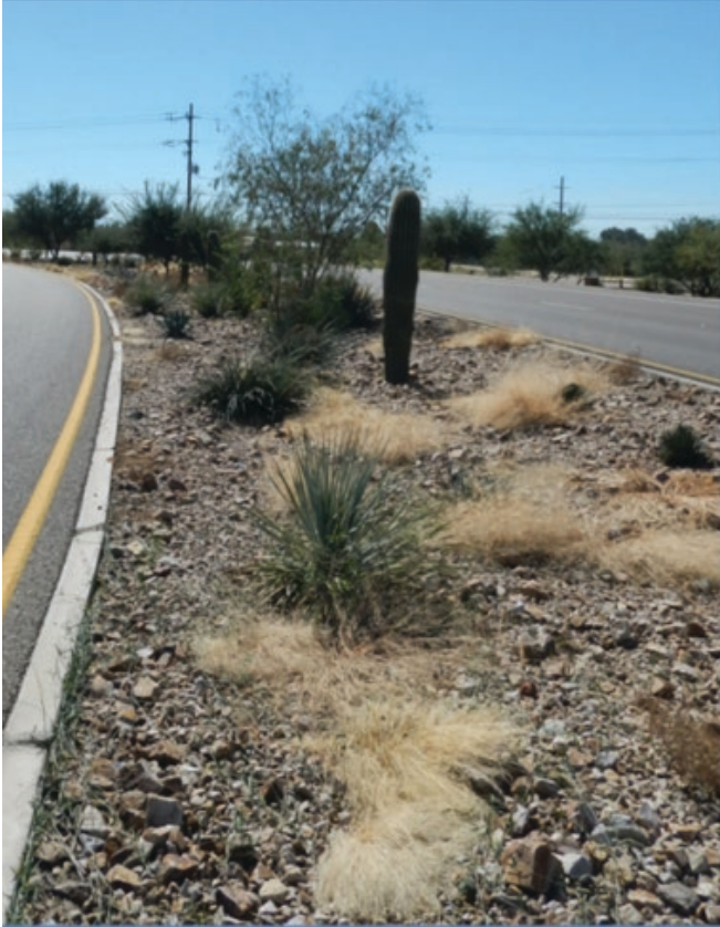
a. Xeriscaping to capture and infiltrate stormwater
