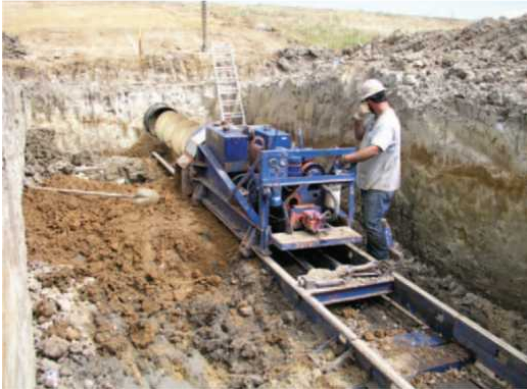
Figure 2-7 - Auger Boring
