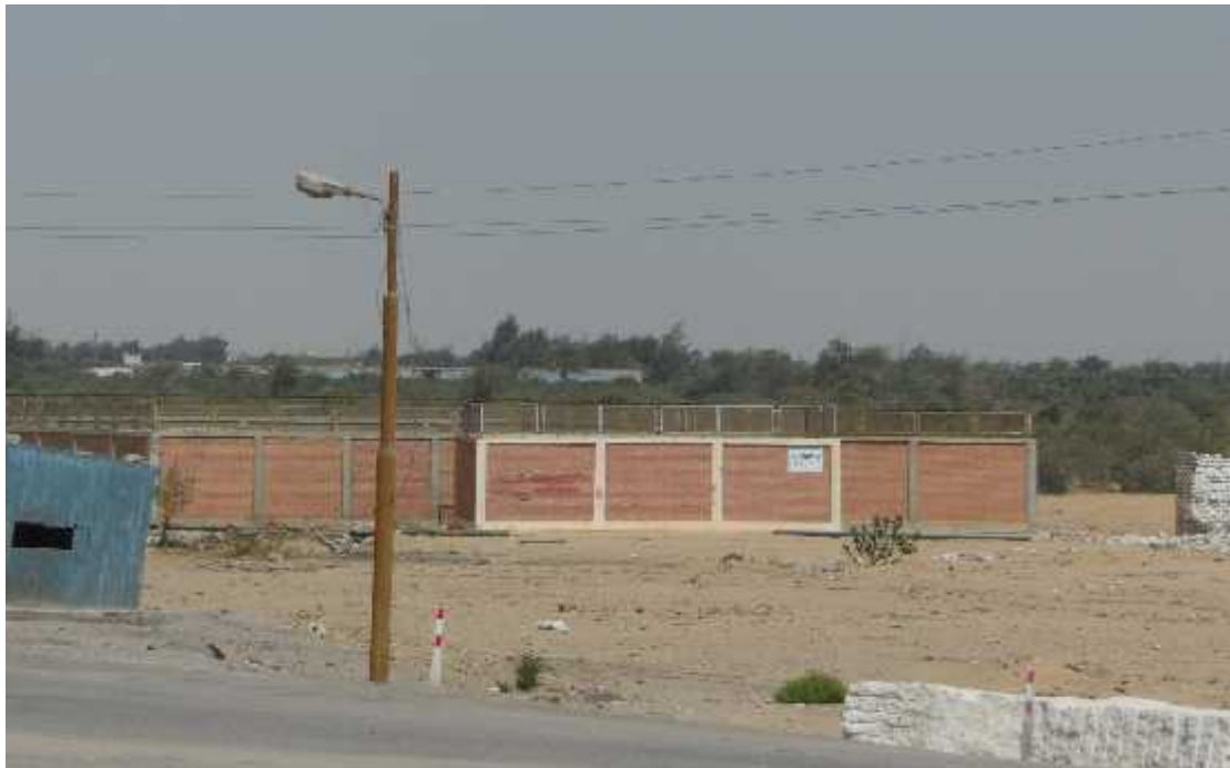
Figure 2-2 - One of the existing valve rooms
