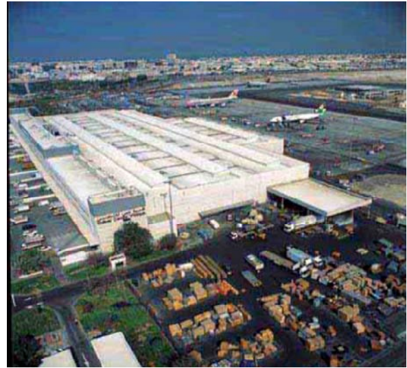
Figure 5-17. Mega Cargo Terminal
