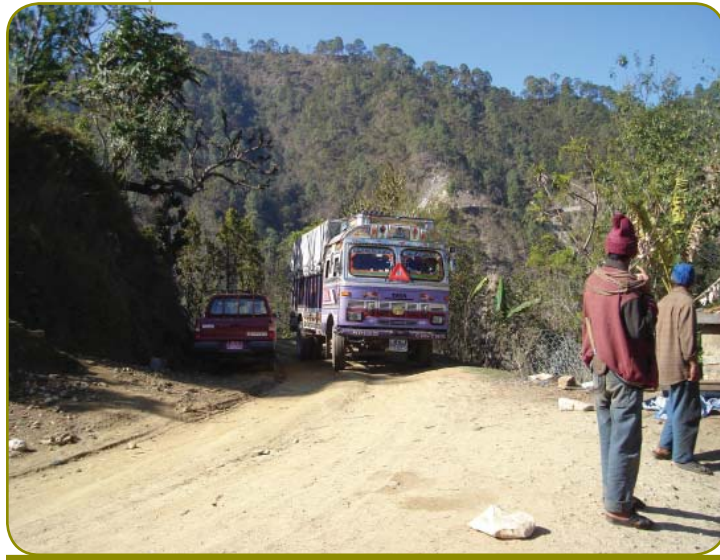
Road on the way to Satbanjh, Nepal. Photo by Marianne Kilpatrick, Senior Transport Specialist, South Asia Sustainable Development Department, The World Bank.
