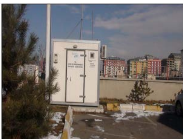
Sample Figure-4: Station photos, Province of Erzurum Air Quality Monitoring Station
