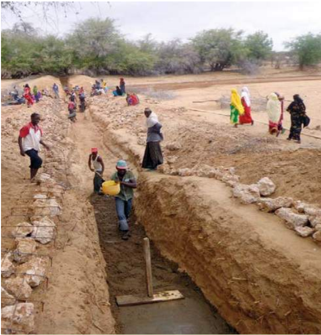
Excavation process (from IUCN archive).
