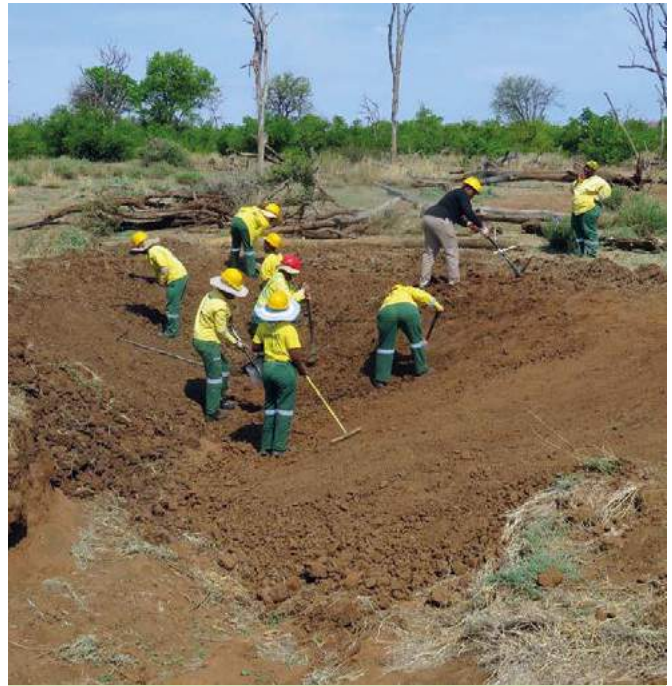
Reshaping of the gully (J Buckle).
