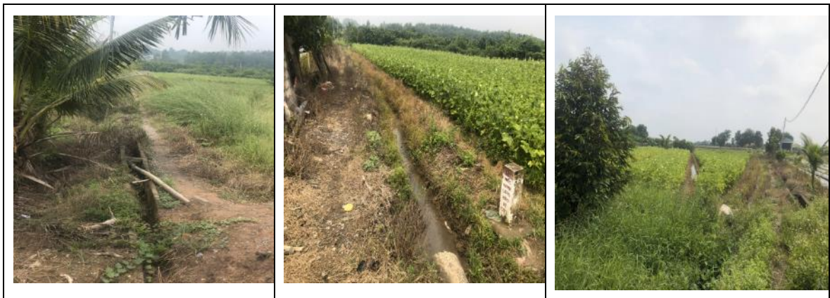
Figure 5.1. Irrigation drains in the at the boundary of Tan Uyen WWTP
