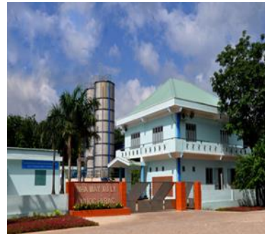
South Binh Duong Solid Waste Treatment Complex
