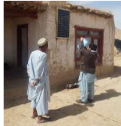
Figure 89 Sub-optimally positioned solar panel in Talkhaki, Samangan
