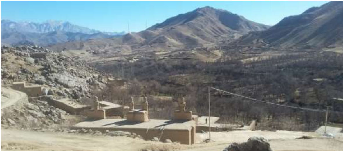
Figure 56 Sang-e-Moom, near Nili, Daikundi. Electricity lines stretch along the valley.
