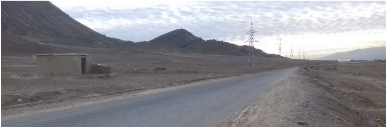
Figure 54 Transmission poles without grid-lines, near to the Gardez Substation in Paktia Province
