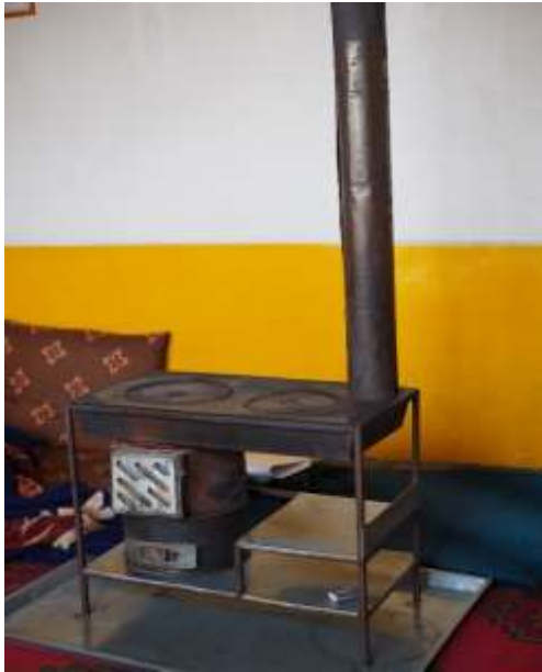
Figure 129 Bukhari wood heater, doubling as a stove to prepare breakfast
