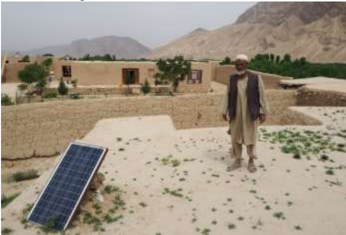
Figure 2 A research participant stands with his solitary solar panel. It charges a battery which powers light-bulbs and mobile phone charging. Talkahki, Samangan
