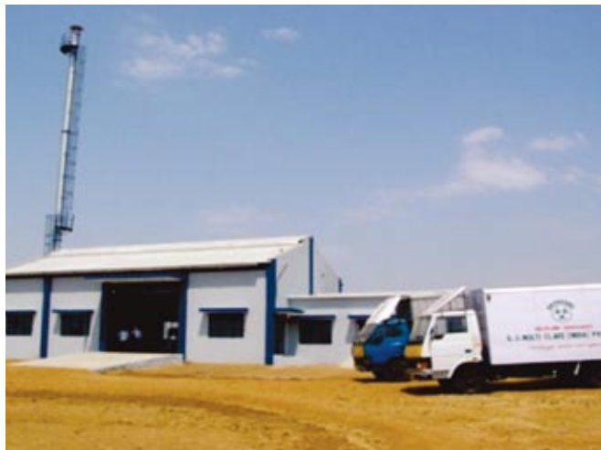
Photo 5.6: Centralized Treatment Facility
