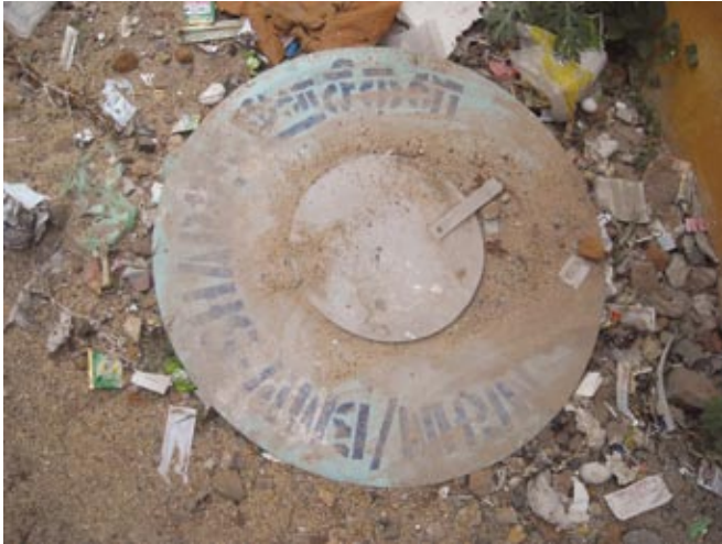
Photo 5.5: Unsatisfactory on-site disposal of health-care waste
