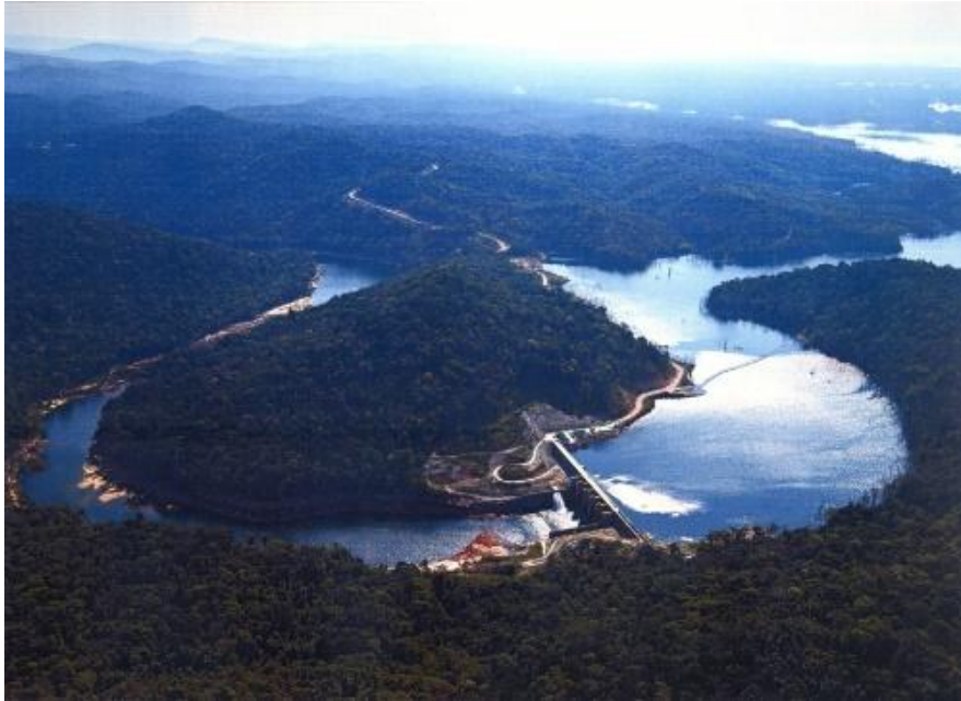
Dam on the Nam Theun, western end of the reservoir (©NTPC/Stanislas Fradelizi)
