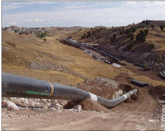
Pipeline construction passes near a hillside community in Turkey.
