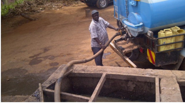
Photo: Emptying fecal sludge at Bugolobi WWTTP. Source: PEAU, Feb 2014
