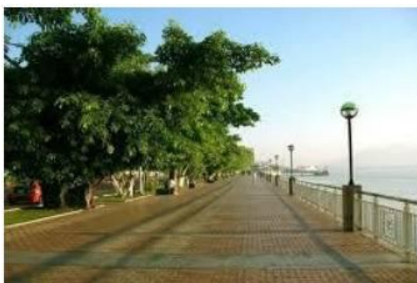
Figure 1.4. Space behind the embankment
