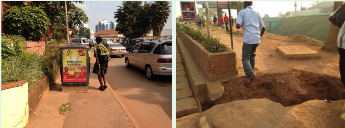
Image 13: Improper street furniture placement (left) and poor maintenance (right) leads to inadequately accessible and obstructed sidewalks.
