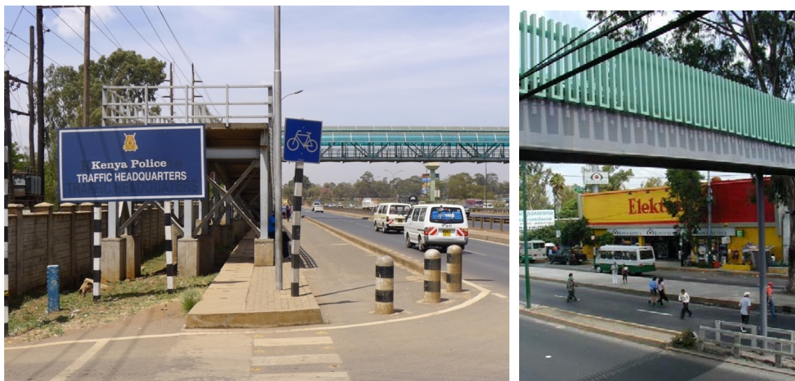
Image 9: Foot overbridges are poor-quality infrastructure that pedestrians often avoid.
