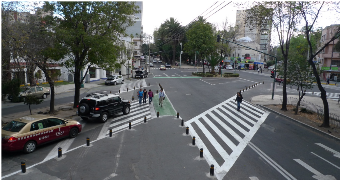
Image 7: Intersection modifications in Mexico City improve pedestrian safety by reducing vehicle lane widths and turning radii.
