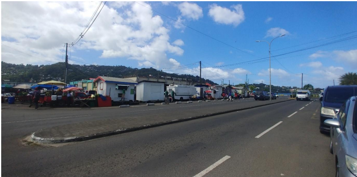
Photo 2 b Sections of Jn. Baptiste Street with a view of the Castries Carpark and the vending huts to be relocated to accommodate the construction of the Box Park
