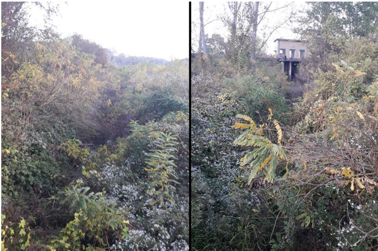
Picture 10. Drainage channel to which impact has been avoided
