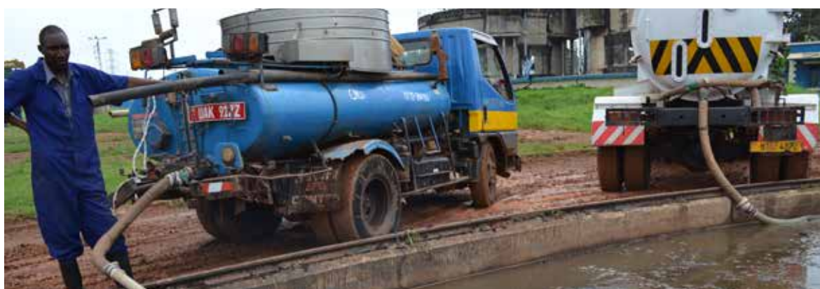
Bugolobi sewage treatment plant. Great Lakes Film Production Ltd (2014)
