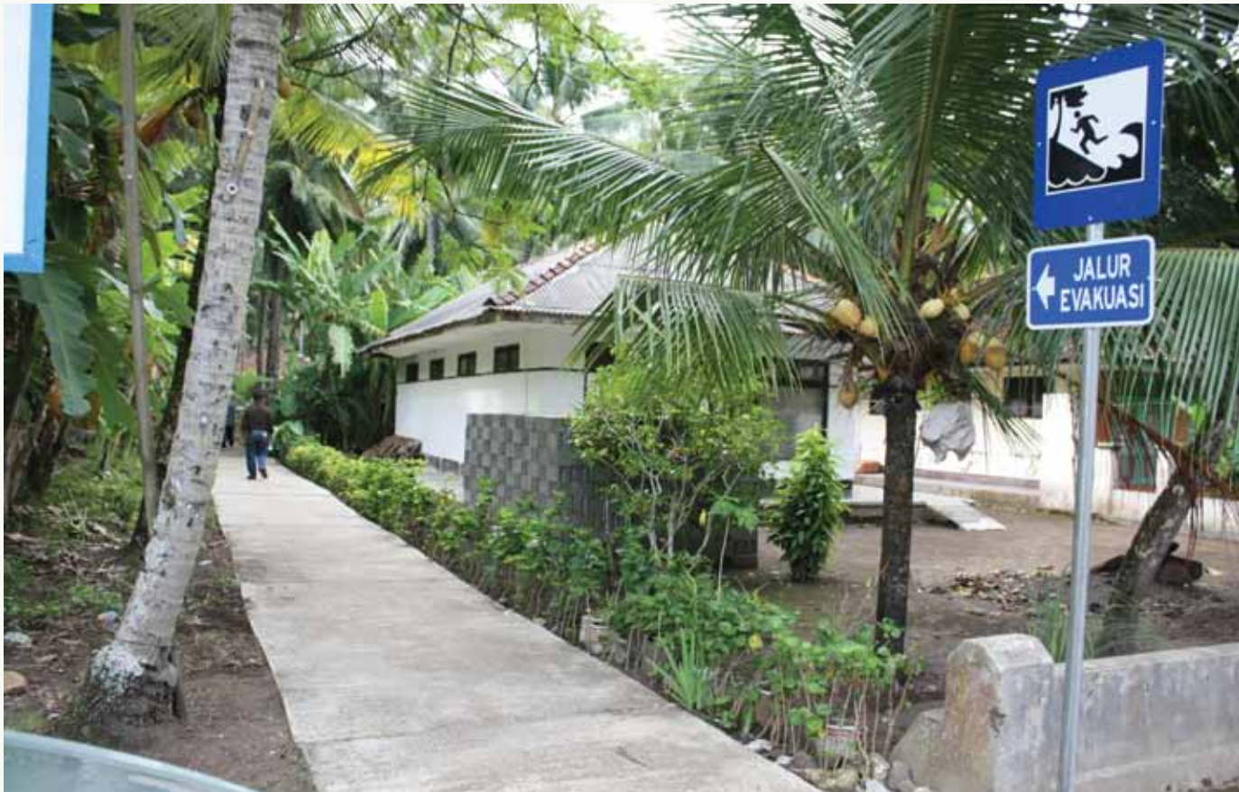
An escape route sign placed near the village road built through Rekompak in Ciamis, West Java, under JRF. Disaster risk reduction measures were an integral part of Rekompak’s community planning process.
