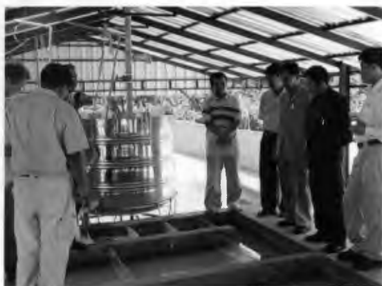
Setting up a treatment facility
