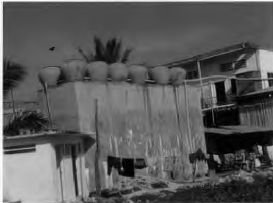
Traditional water tower
