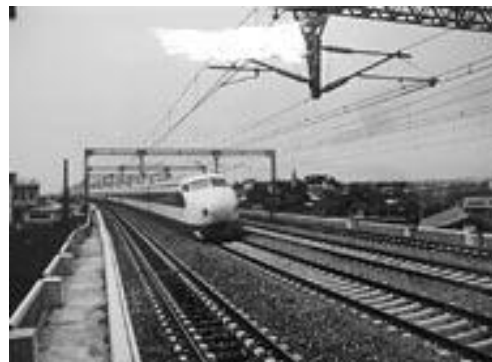
A view of an embankment on the Tokaido Line
