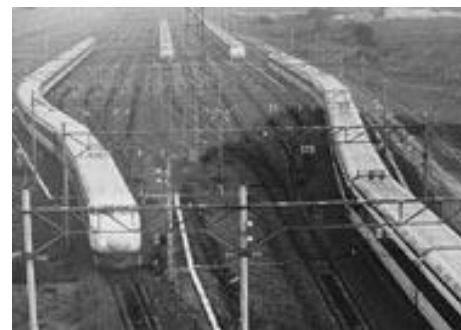
The new train depot and fitting out station at Torikai rail station, between Osaka and Kyoto
