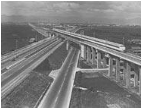
The new double track wide-gauge line runs parallel with the old narrow-gauge line from Tokyo to Osaka. The new line will be used only for express passenger and express freight trains, reaching speeds of 125 miles an hour
