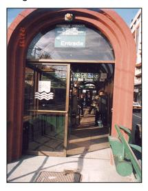
assist those who are unable to walk long distances. An exit should be considered at the "far end" of stations even if an entrance is not possible. Exit doors should provide a minimum of 900 mm of clear space. Manually operated doors should open easily, requiring no more
