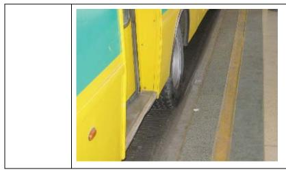
The use of a beveled curb at bus stops may enable drivers to position their buses closer to the curb by bringing the front tire into safe contact with the curb. This can greatly reduce the combined horizontal and vertical distances which passengers must overcome to reach the first step of the bus.
