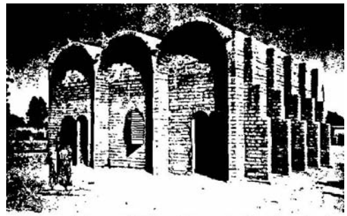
Figure A3.4 Earth-built School in Niger (1986–87) by MoE with World Bank Assistance
