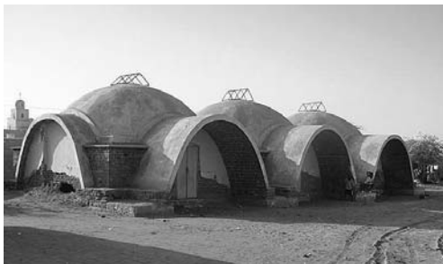
Figure A3.2 Rosso (Mauritania) 1979: School Built with Earth and Vault Technology by the NGO ADAUA
