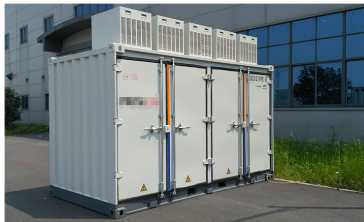
c. Ventilation units raised above the battery energy storage system
