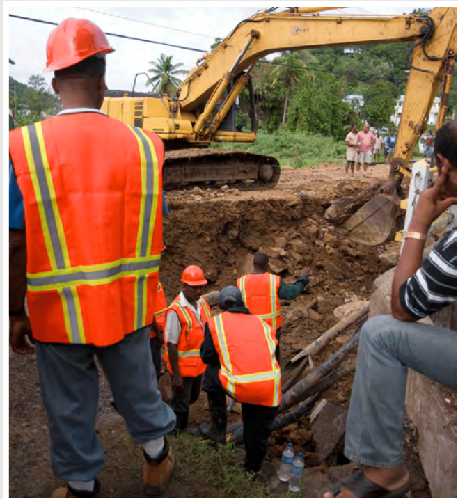
Workers in St. Lucia repairing damaged bridge from Hurricane Tomas. Photo: © jaminwell.
