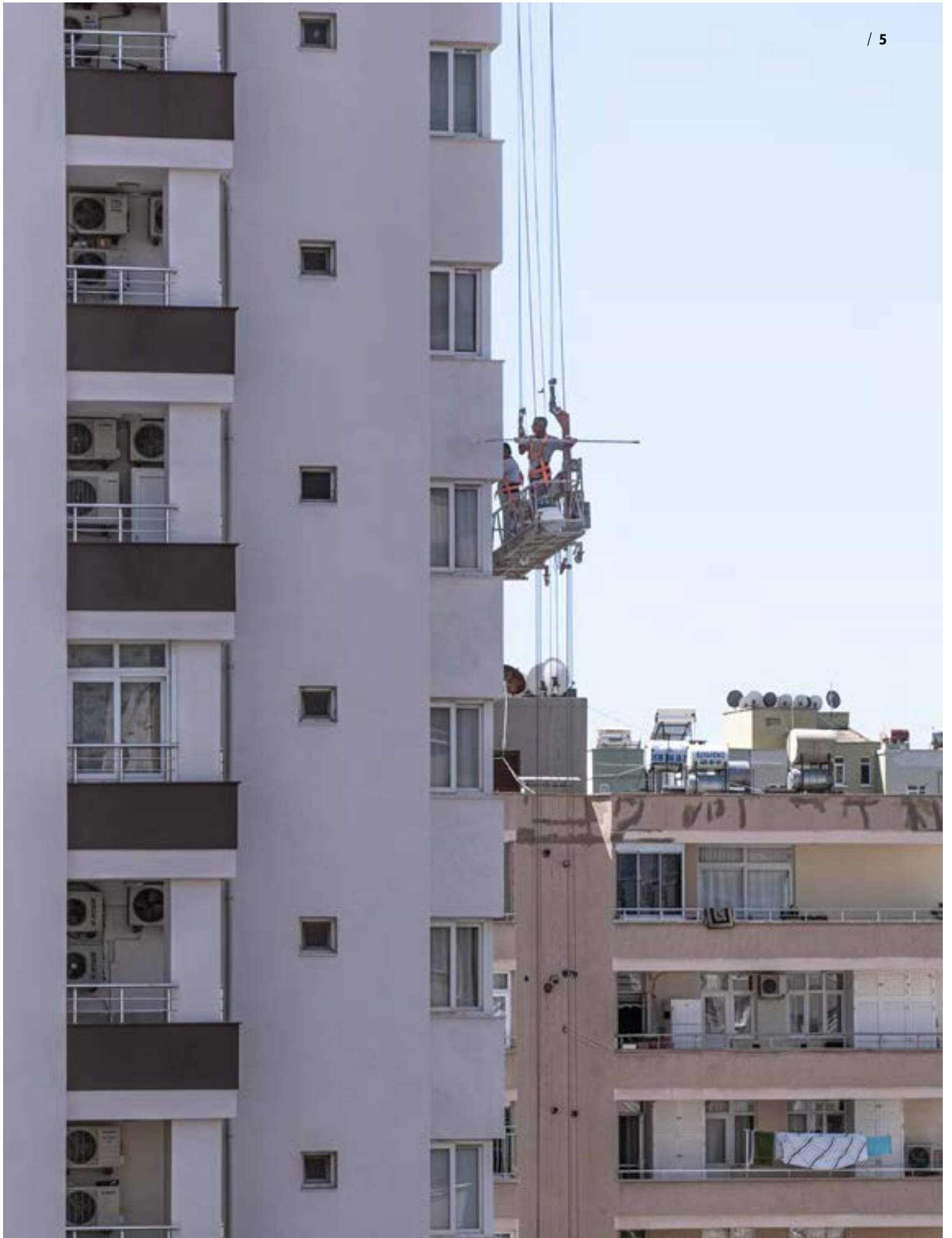
June 2023 repairs of slightly damaged buildings in Adana, Turkey. Photo: © mustafaoncul.
