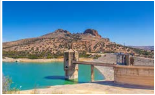
Sidi Salem Dam, Tunisia's largest dam, on the Medjerda River. Photo: © Khaled Ladjimi.
