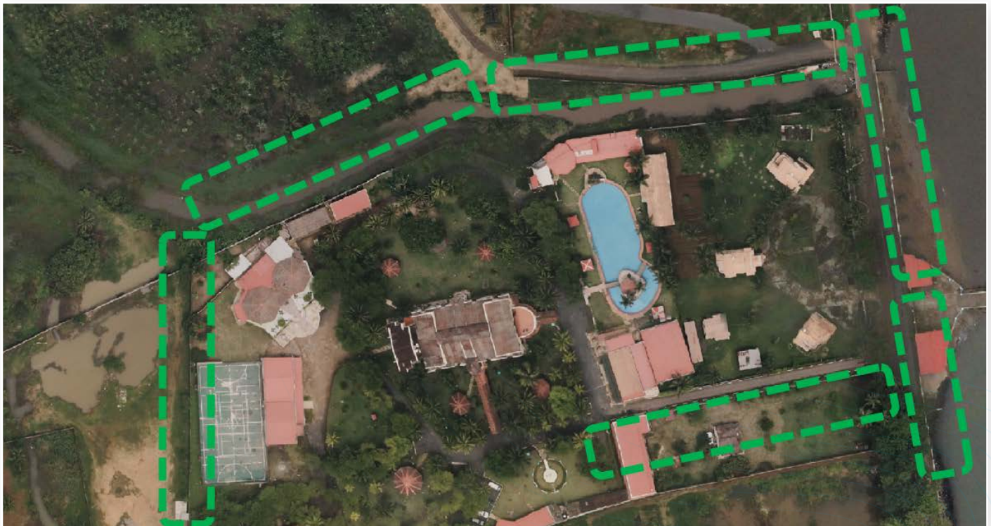
A high-resolution aerial photo (20cm pixels) around Hotel Praia, showing the “network” of coastal and fluvial protection walls marked in green. Source: Abnilde Ceita Lima/WACA PIU
