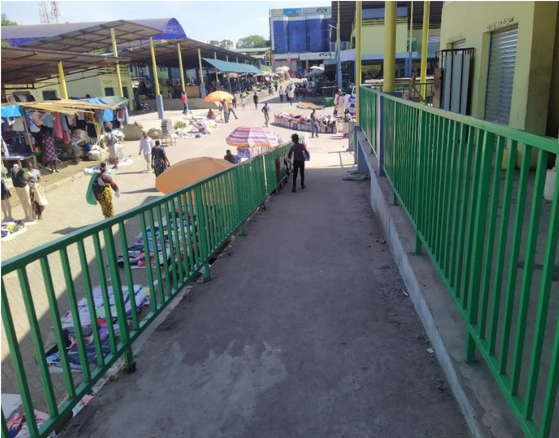
Figure 5. Good practice in universal access: A wheelchair accessible ramp at the Homa market
