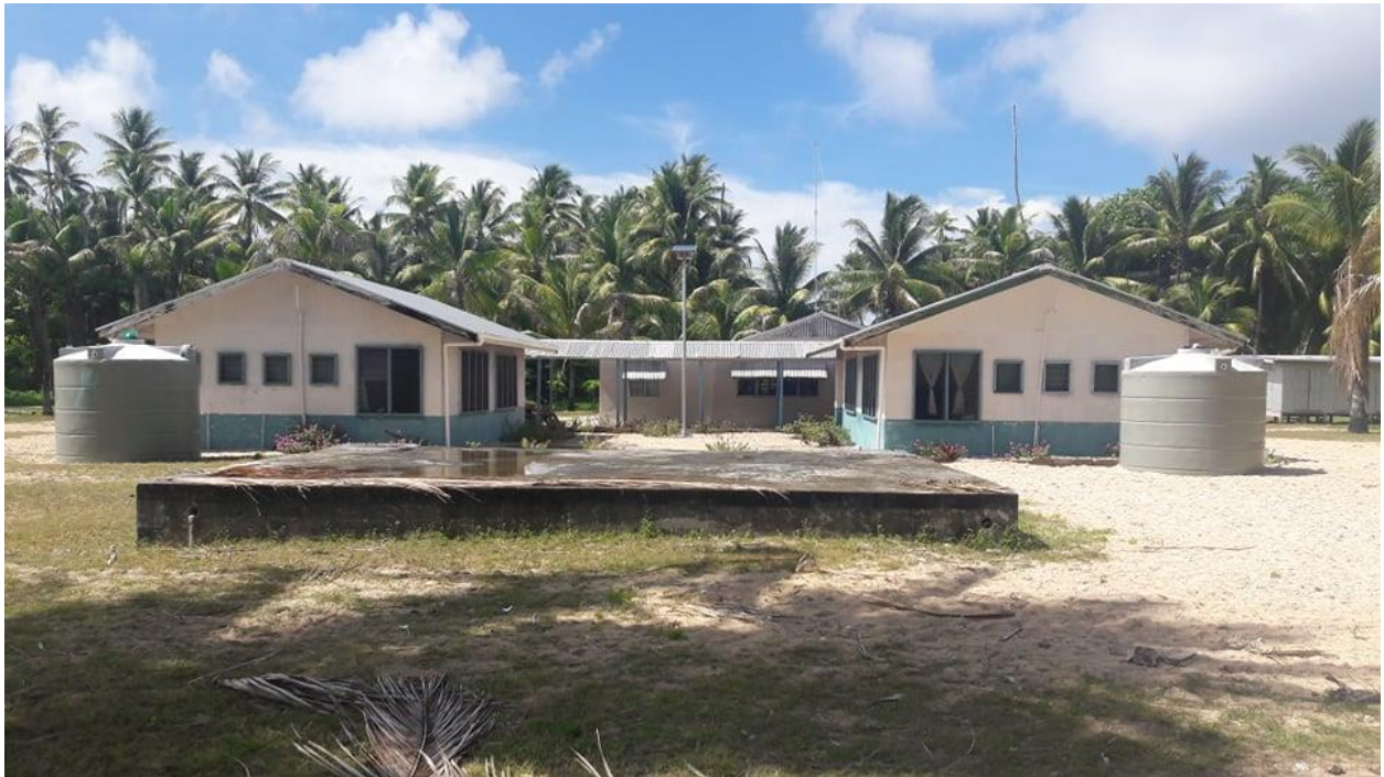
Figure 14: Eastern side of Nui Clinic
