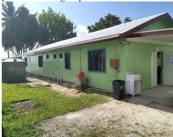
Figure 2: Clinics adjacent to Project site (North) site (East)
