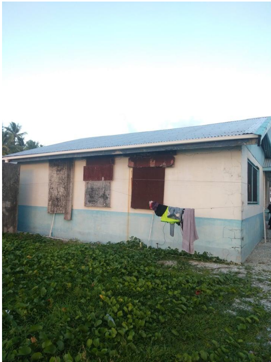
Figure 35 West side of the clinic
