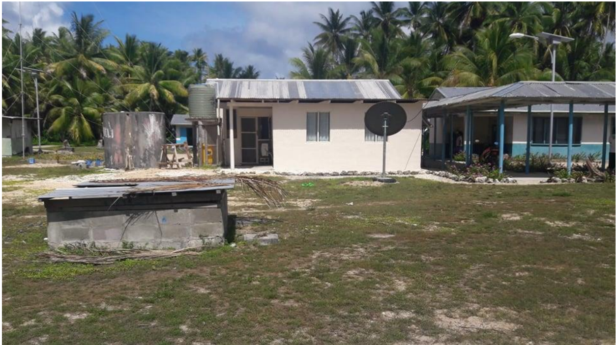
Figure 16: Southern side of Nui Clinic
