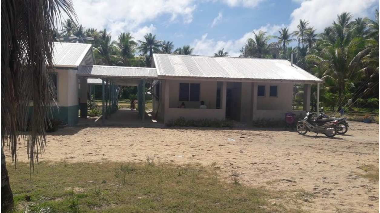
Figure 13: North side of Nui Clinic
