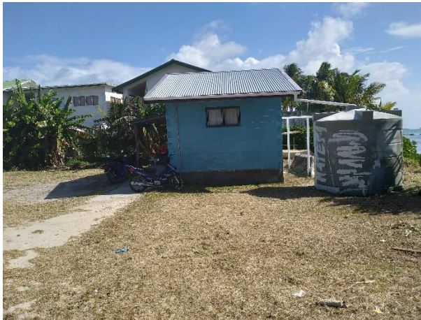
Figure 6: Oxygen room adjacent to project site (West) project site (West)
