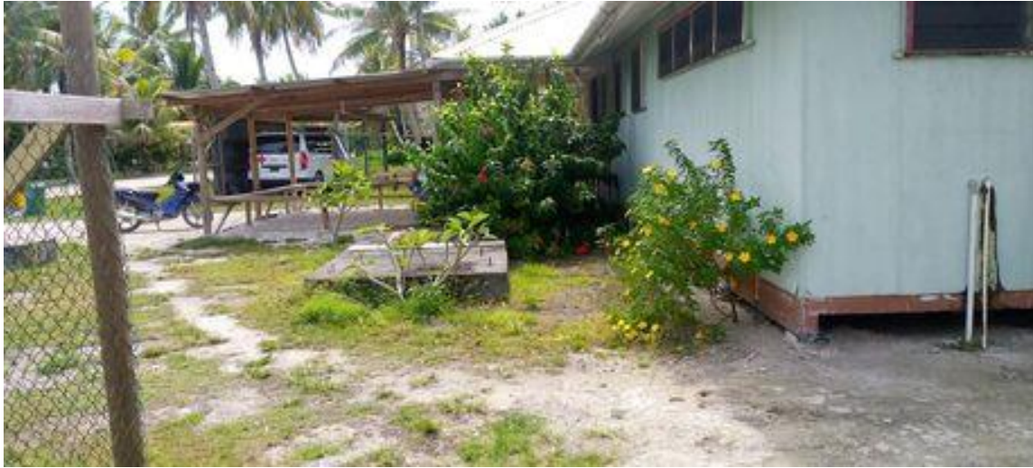
Figure 17: Eastern side of Vaitupu Clinic
