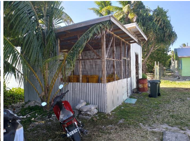
Figure 7: Waste storage room adjacent to project site (West)
