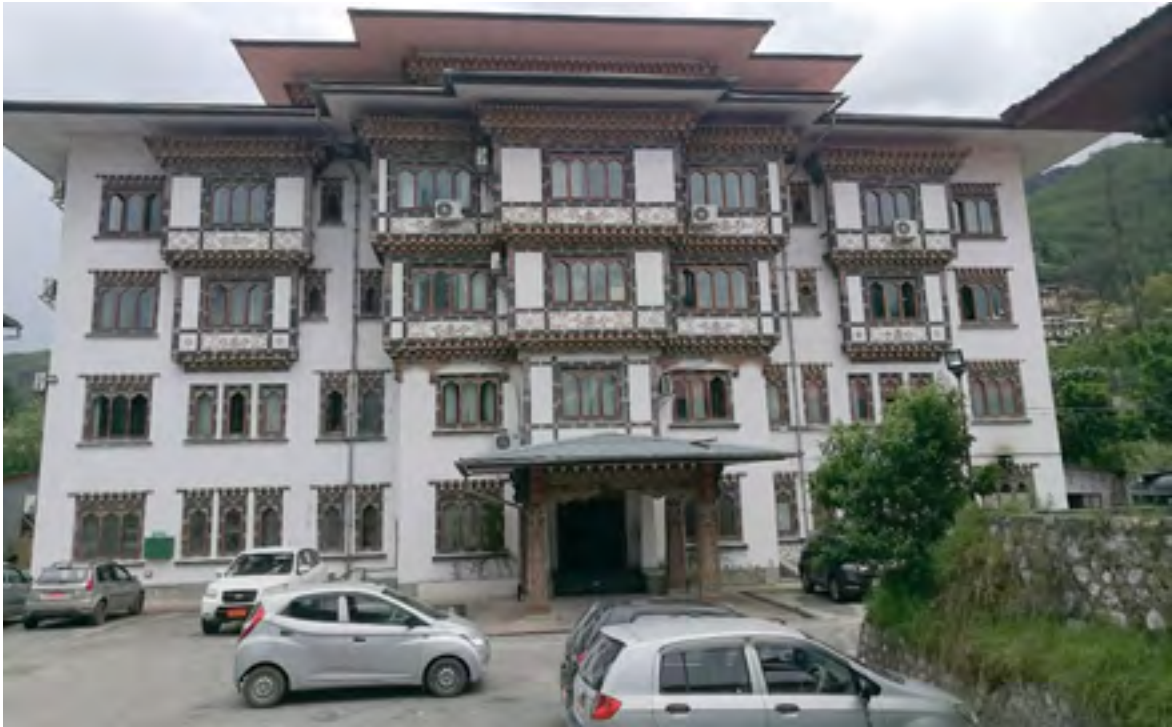
Figure ES.4. The Headquarters building of NCHM is shared with other government agencies
