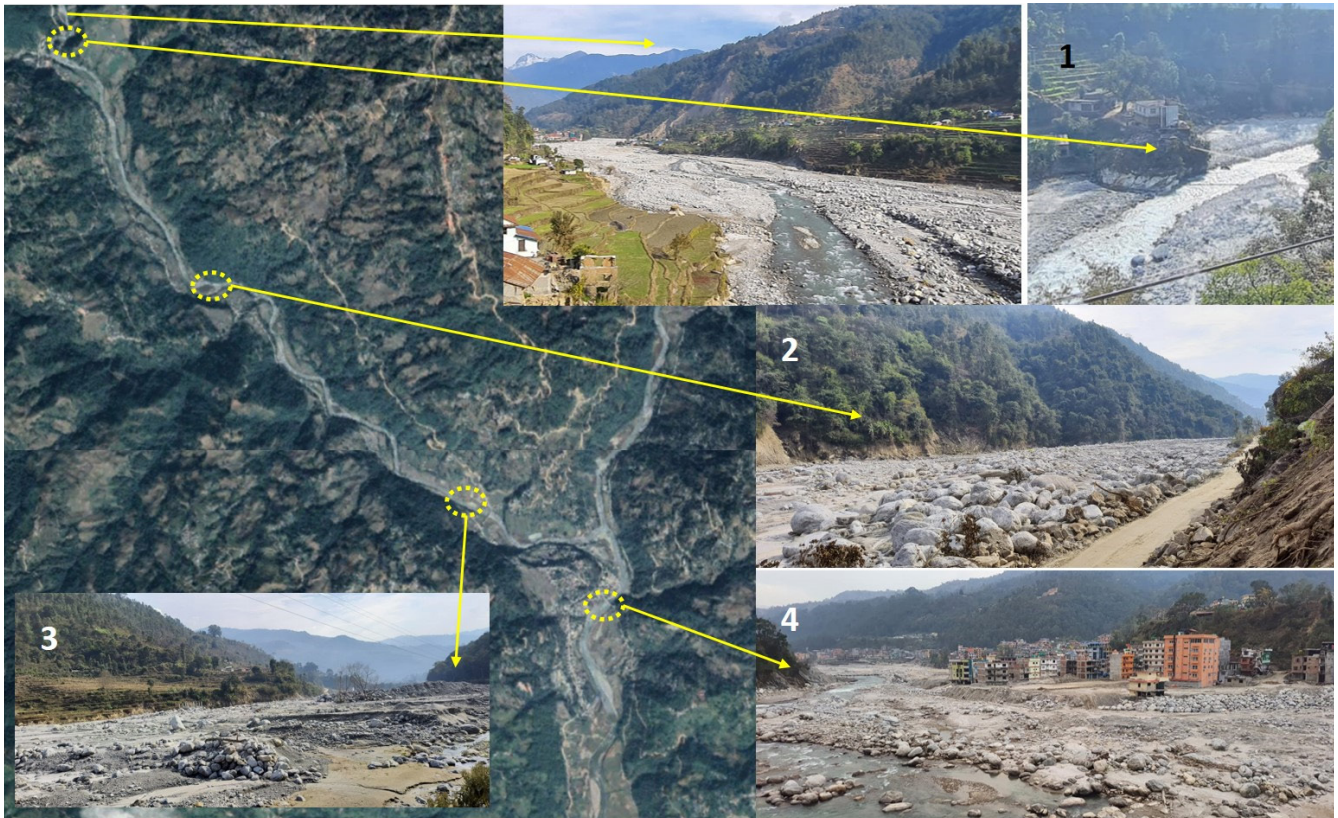
Figure 23: Four locations (Talarang to Melamchi Bazar section) of sediment blockage during the 2021 flood in the Melamchi River. These locations highly controlled the sedimentation process. Location 1 is Talarang, location 2 is Thulophat, location 3 is Phatte, and location 4 is Melamchi River.
