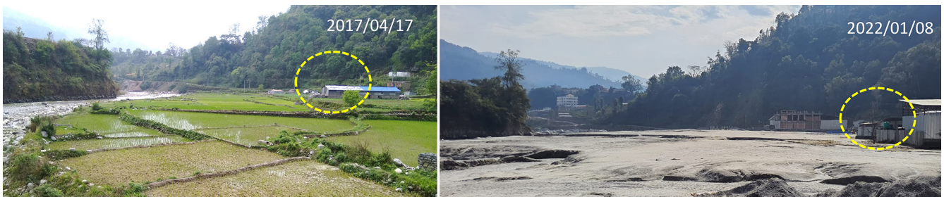
Figure 24: Significant deposition of debris occurred at Phatte due to a slowdown of flow caused by a downstream bridge as a blockage. Only fine sediments were found deposited downstream of the bridge.
