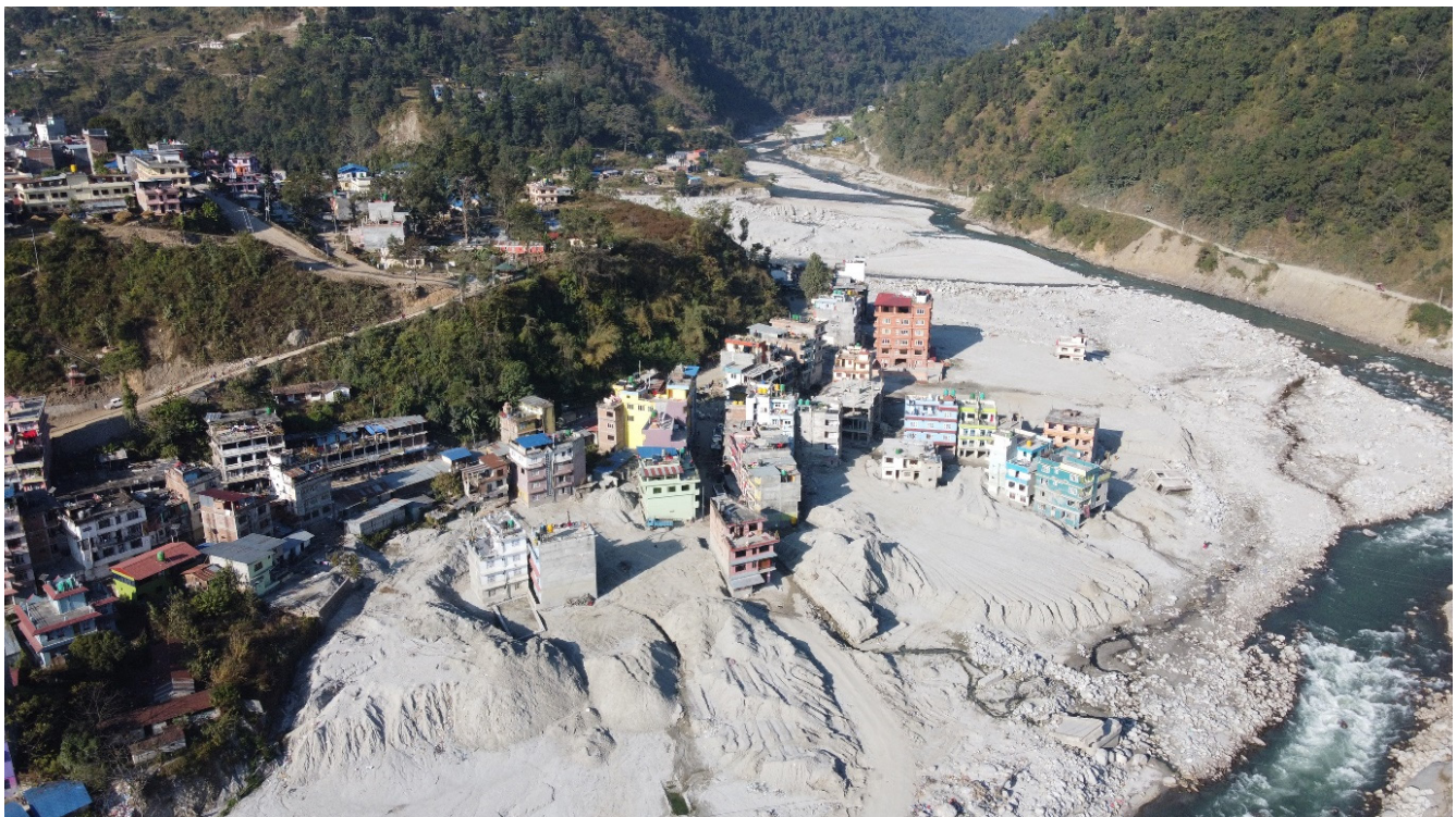
Figure 26: Many buildings in Melamchi Town was covered by the debris.
