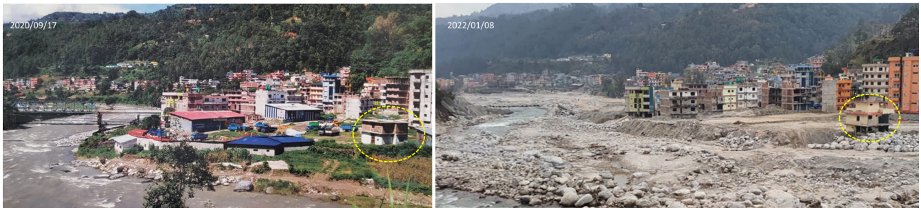
Figure 25: Before and after view of damaged Melamchi Bazar. The Pul Bazar was the major obstacle, and more than 16 m of sediment was accumulated in the Melamchi Bazar.
