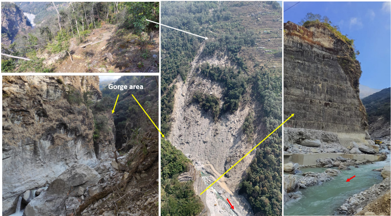
Figure 22: Landslide in headworks area, deep gorge and headworks area under cleaning.
