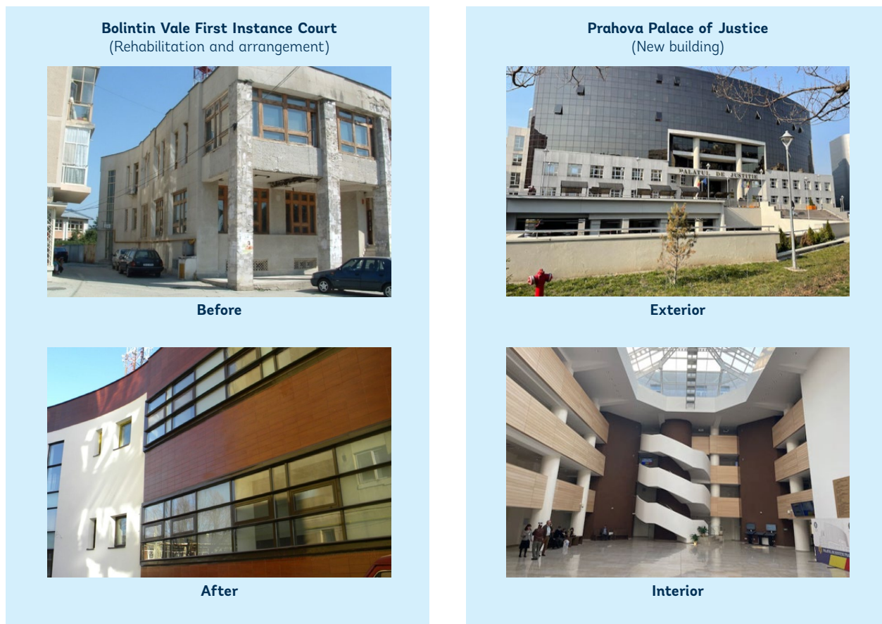
FIGURE 9. Examples of recent investments in justice infrastructure
