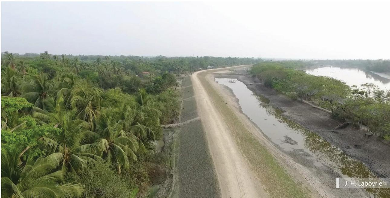
Example of coastal embankment and turfing (Polder 35/1).
