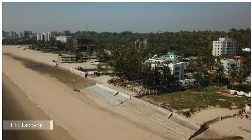
Short seawall with mild slope and crest accessible by stairs.
