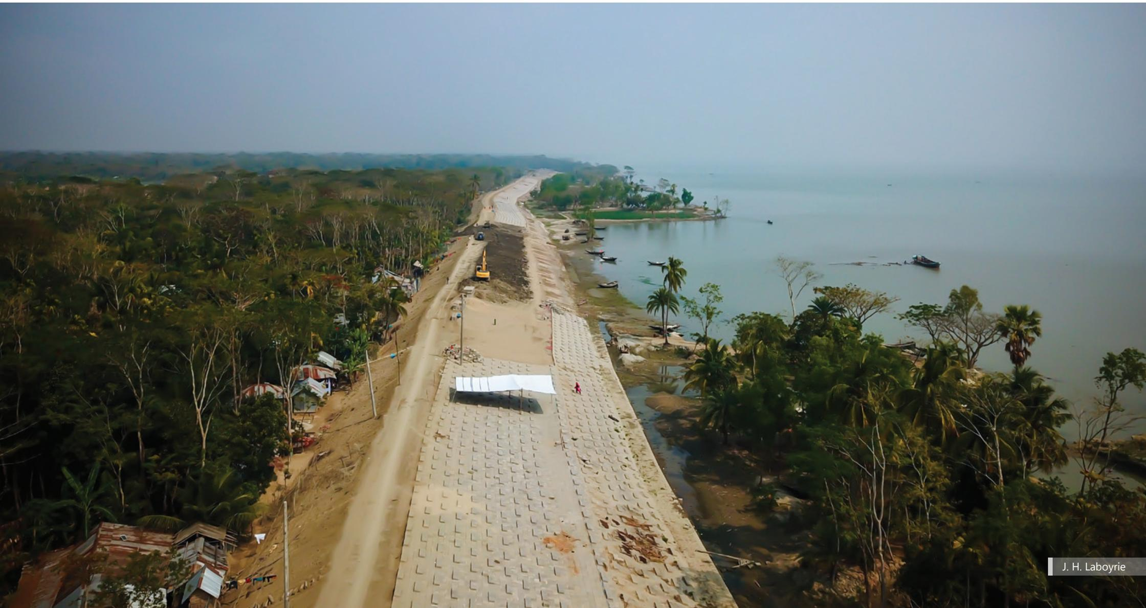
Example of coastal embankment slope protective works in Polder 35/1.
