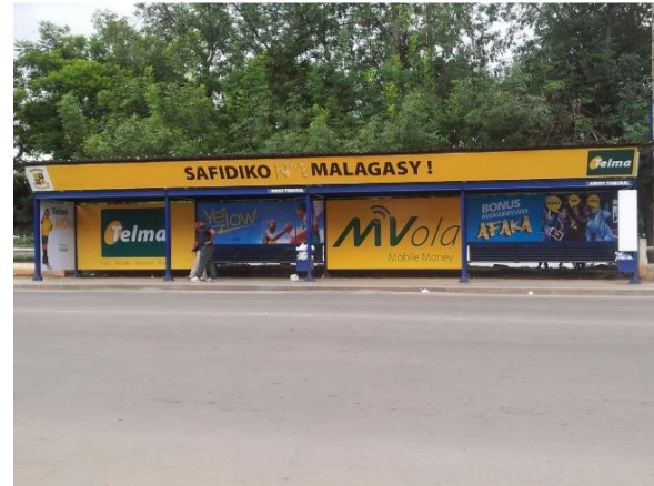
Figure 39. Bus Station in Antananarivo
