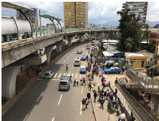
Figure 2. Sidewalks around the LRT Corridor.
