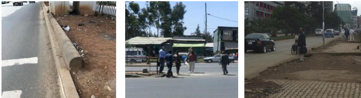
(a) Lack of sidewalk or deficient construction and design (b) Presence of guard rail and illegal crossings (c) Construction and maintenance deficiency, and pedestrian invasion of the road
