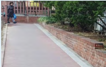
Lack of safety handles; pedestrian walkway not separated from surroundings.
