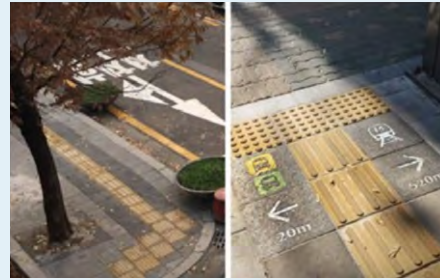
Pedestrian obstacles removed; ground leveled; sidewalk blocks and floor guides with varying degrees of contrast provided for those with poor vision.
