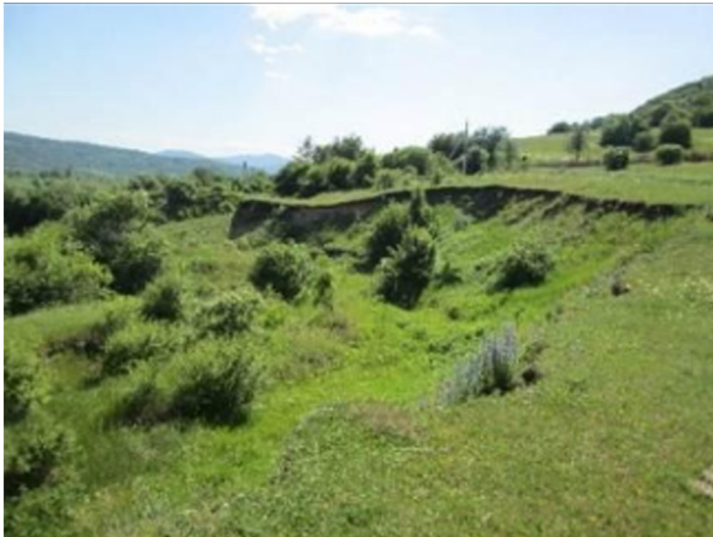
Figure 20. Active landslide on the right slope of the Sagami River valley 22
