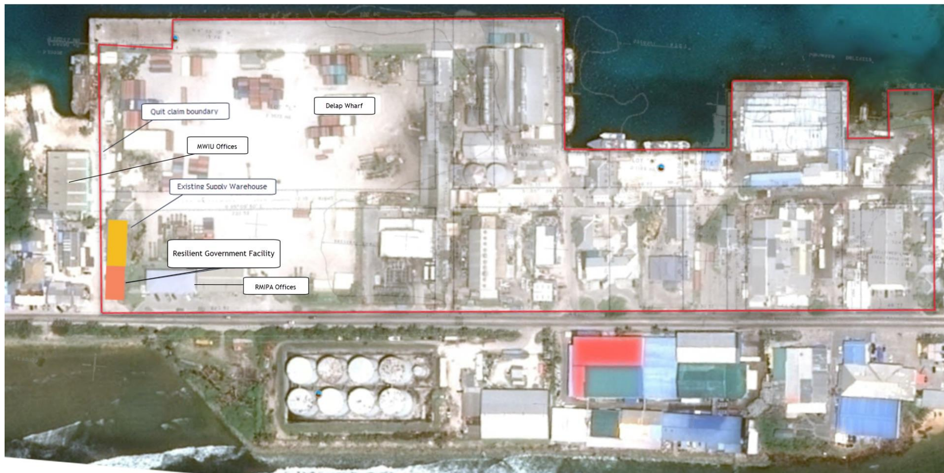
Figure 15: Resilient Government Facility site layout showing area covered by quit claim (in red) and existing neighboring buildings
