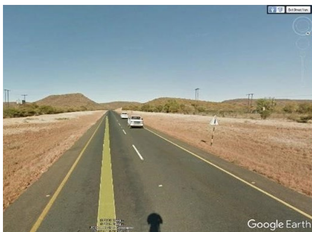
PBC area (before Rehabilitation)
