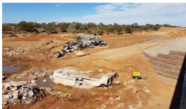
FIGURE A4.45: EMERGENCY WORK REINSTATEMENT FOLLOWING FLASH FLOOD
