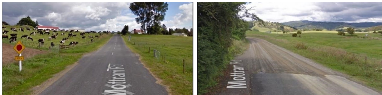
FIGURE A4.22: TYPICAL PAVED RURAL ROAD SERVING AN INTENSIVE DAIRY INDUSTRY AND PAVED TO UNPAVED RURAL ROAD TRANSITION
