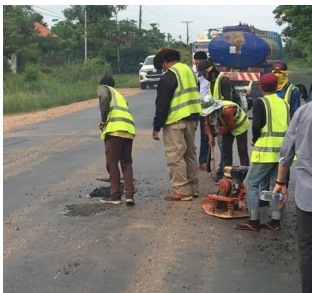
FIGURE A4.8: POTHOLE REPAIRS UNDERTAKEN UNDER A TRADITIONAL CONTRACT
