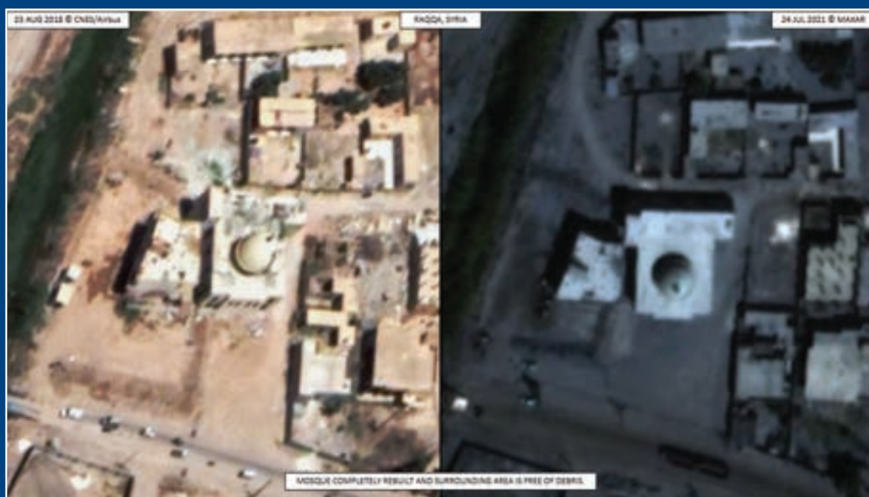
Example of a facility classified as No Damage.
