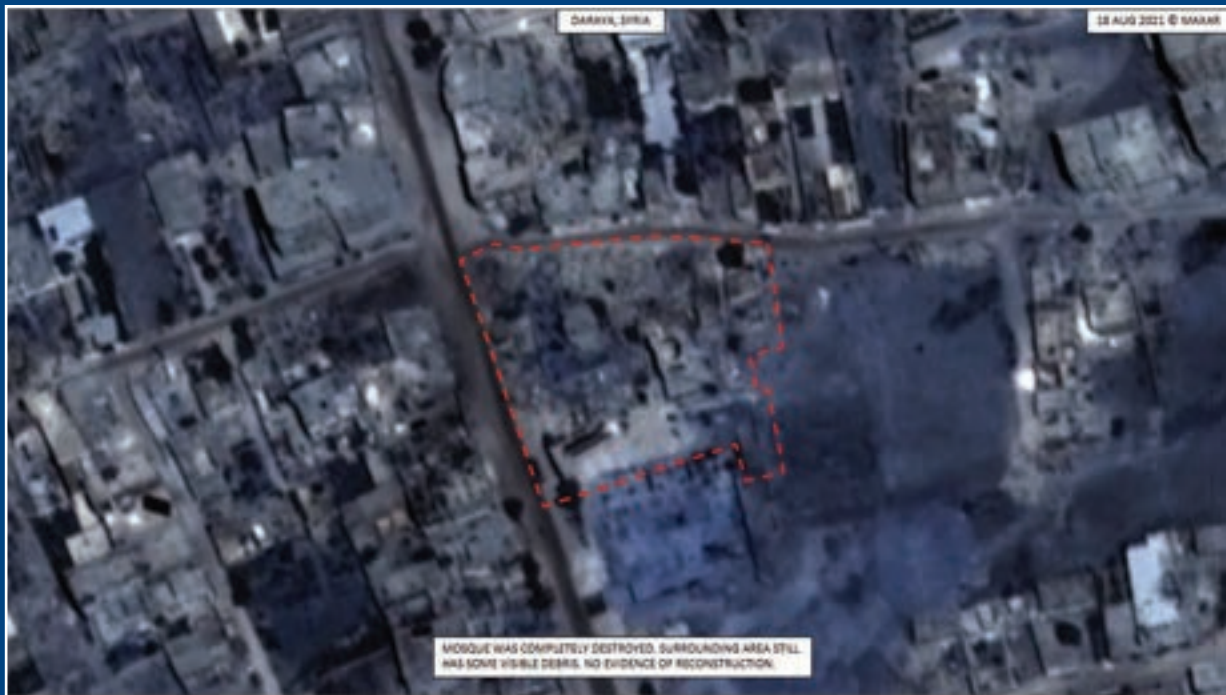
Example of a facility classified as Destroyed.
