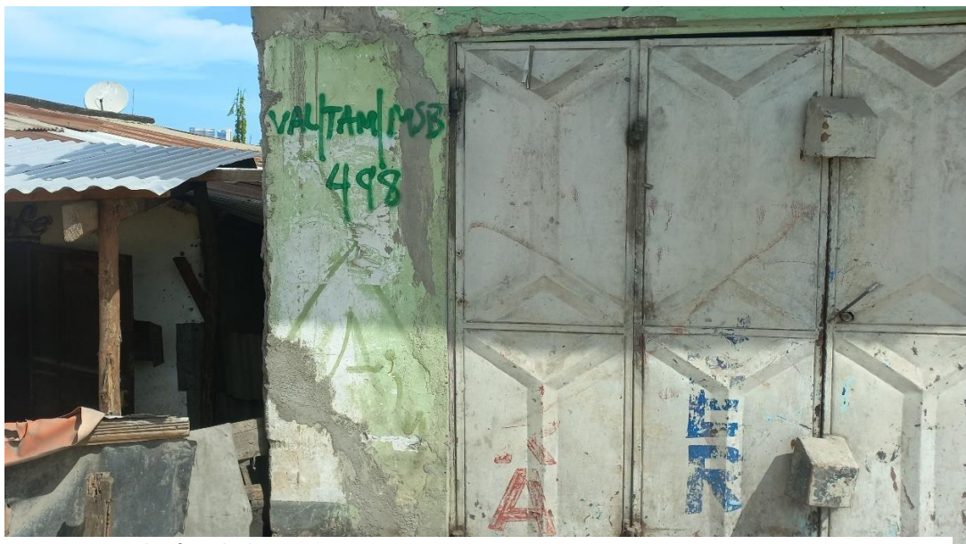
Figure 7-1: Example of marked structure
