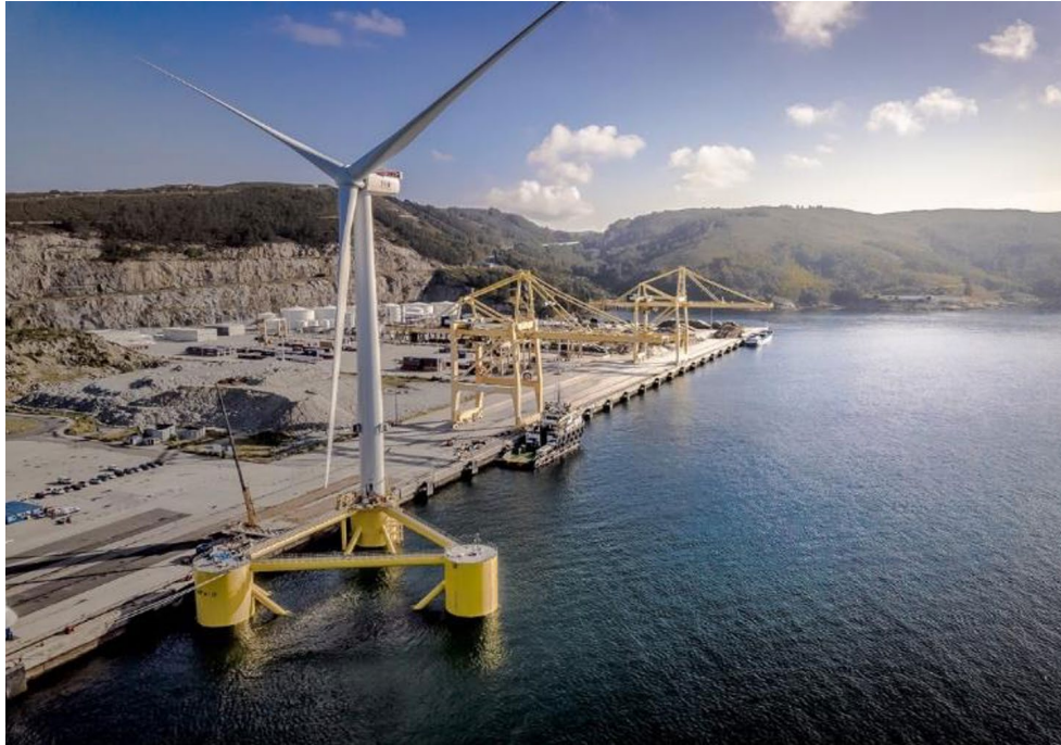
FIGURE 11.5 WTG MOUNTED ON A SEMI-SUBMERSIBLE FOUNDATION FLOATED DIRECTLY AT QUAYSIDE [79].
