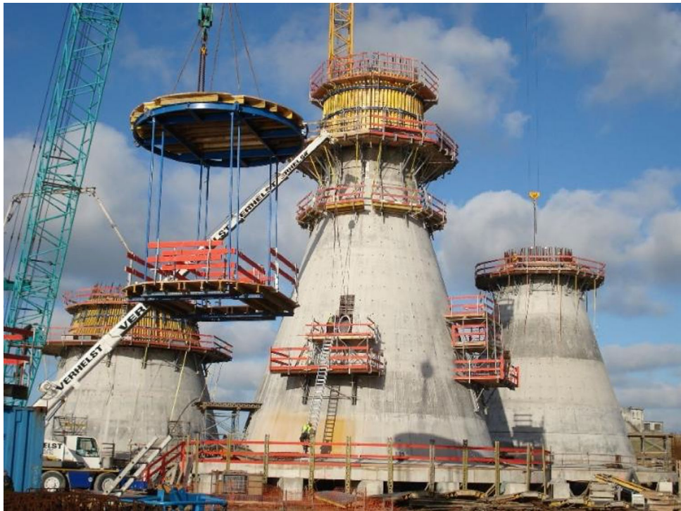
FIGURE 12.6 GRAVITY-BASED FOUNDATIONS FOR THORNTON BANK (SOURCE: COWI).
