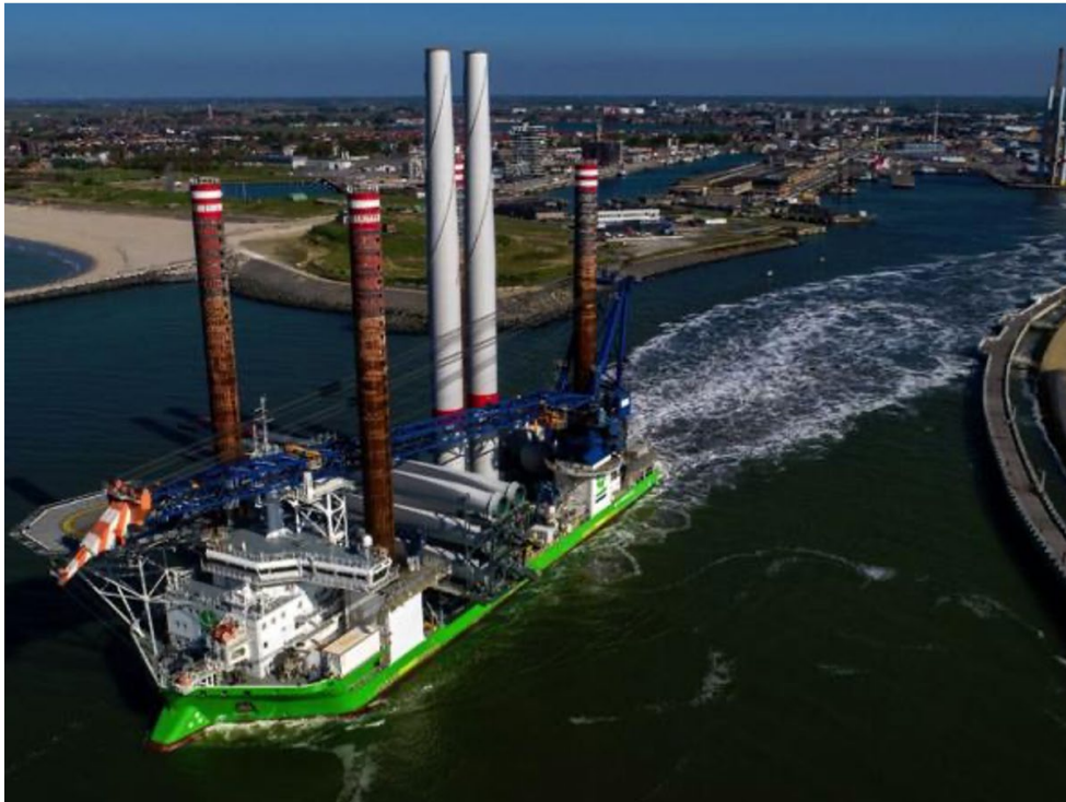
FIGURE 11.1 WTG INSTALLATION VESSEL AT SAIL AWAY FROM HARBOR [76].
