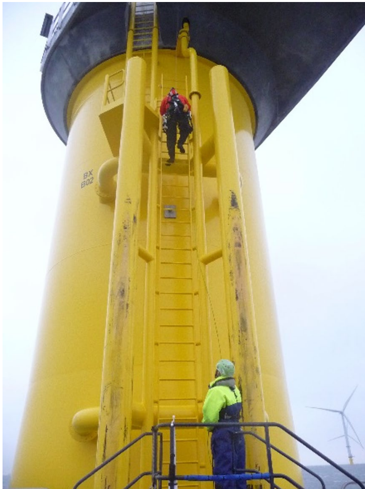
FIGURE 12.11 OFFSHORE WTG TECHNICIAN ACCESSING A WTG (SOURCE: COWI).
