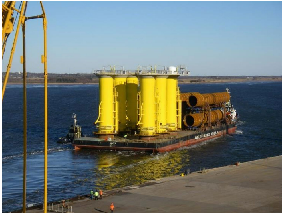
FIGURE 12.7 MONOPILES AND TRANSITION PIECES AT SAIL AWAY FOR LONDON ARRAY (SOURCE: COWI).
