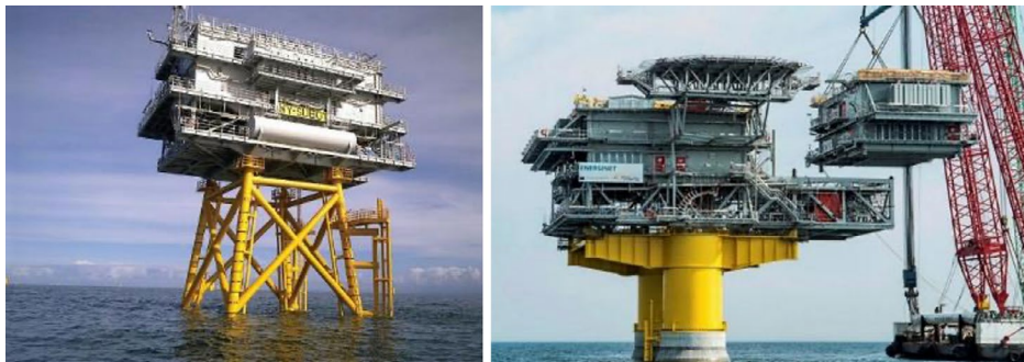
FIGURE 12.9 OSS OF OWF WALNEY EXTENSION (LEFT) ON JACKET FOUNDATION AND OSS OF OWF KRIEGERS FLAK ON MONOPILE (SOURCE: COWI).
