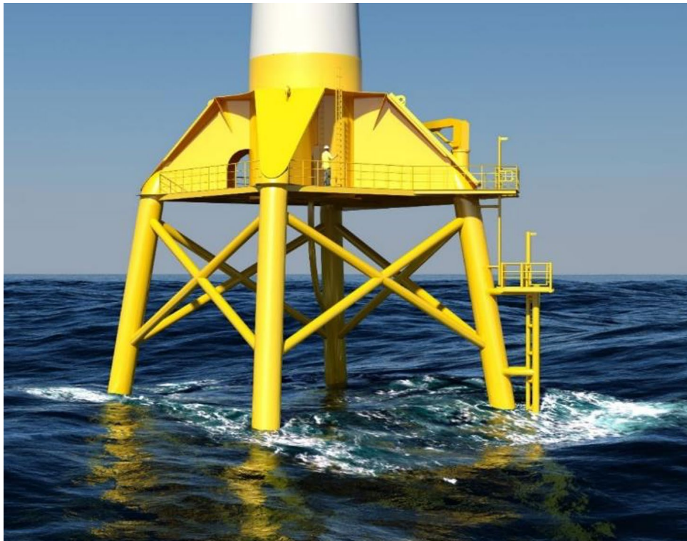
FIGURE 12.8 JACKET STRUCTURE AT WIKINGER (SOURCE: COWI).
