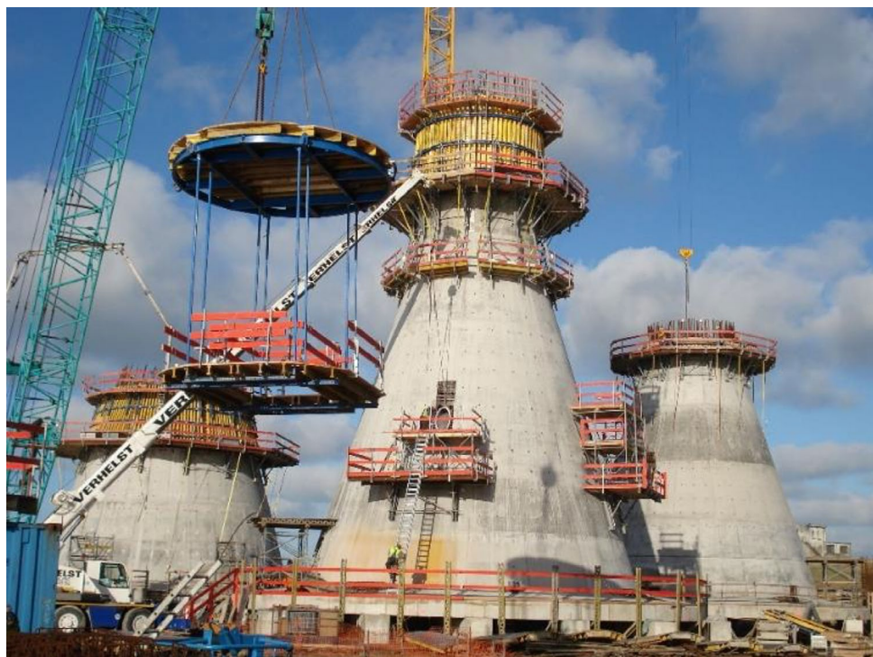
FIGURE 12.6 GRAVITY-BASED FOUNDATIONS FOR THORNTON BANK (SOURCE: COWI).
