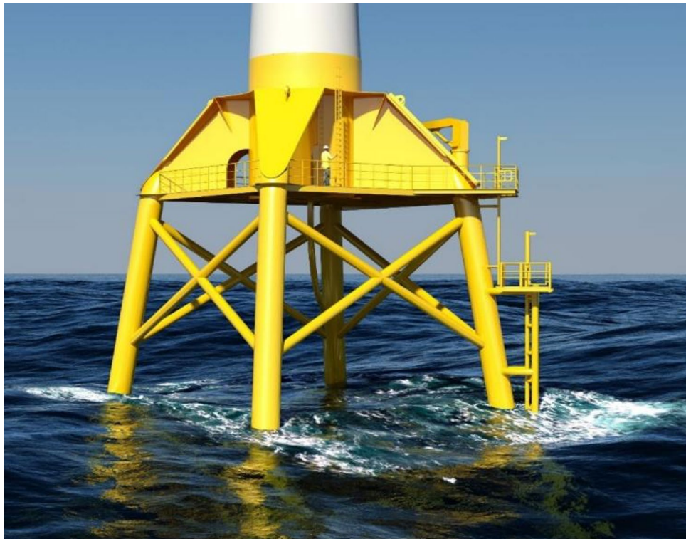
FIGURE 12.8 JACKET STRUCTURE AT WIKINGER (SOURCE: COWI).
