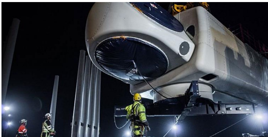
FIGURE 12.5 THE MASSIVE ROTOR HUB AND NACELLE OF A VESTAS 164-9.5 MW BEING LIFTED TO A VESSEL [91].
