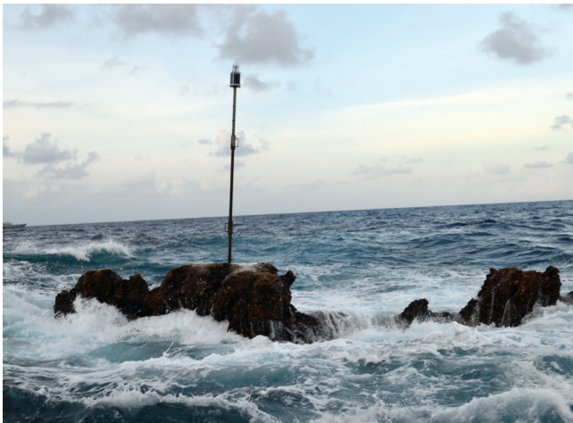
Figure 10. Low tide elevation with navigational aid installation
