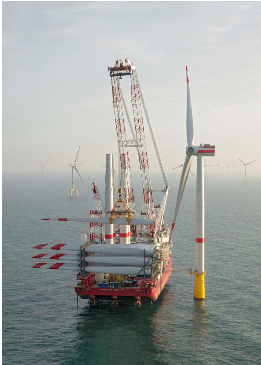
FIGURE C7.5 EXAMPLE TURBINE INSTALLATION VESSEL
